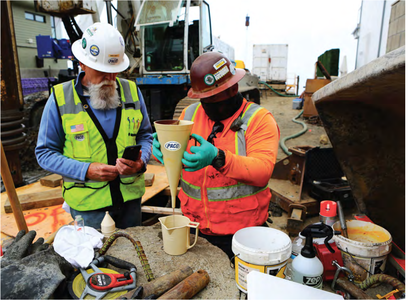
SLURRY ENGINEER MIKE HAGY SUPERVISING THE SLURRY PREPARATION
